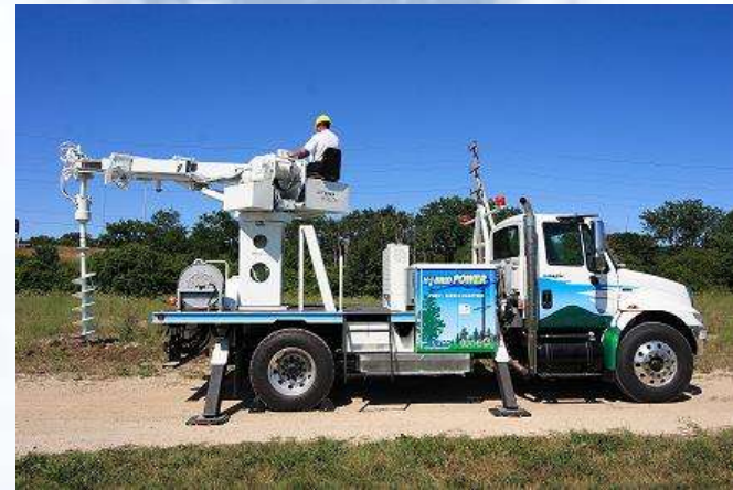
Hybrid Digger Derrick
