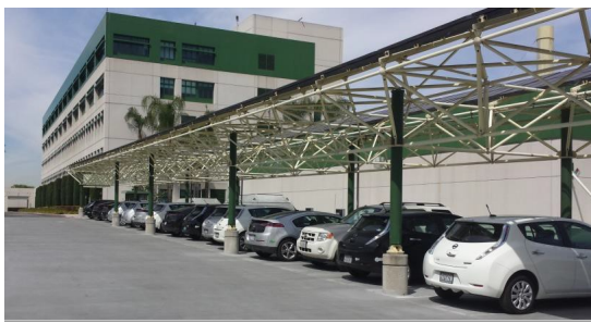
Level 2 Chargers Under Solar Carport
