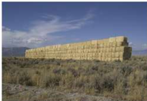
Fig. 3. Mock straw bale noise barrier, 6 m high and 20 m long.
