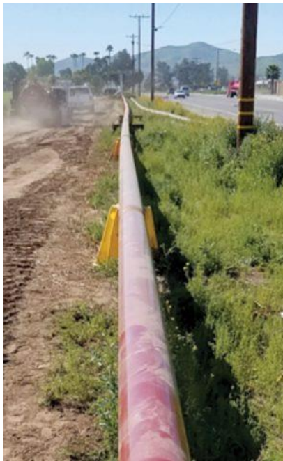
Figure 4. Biogas transported with the 1.4-mile pipe (left) and SoCal gas point of receipt (right), Photo courtesy of CR&R Waste and Recycling Services
