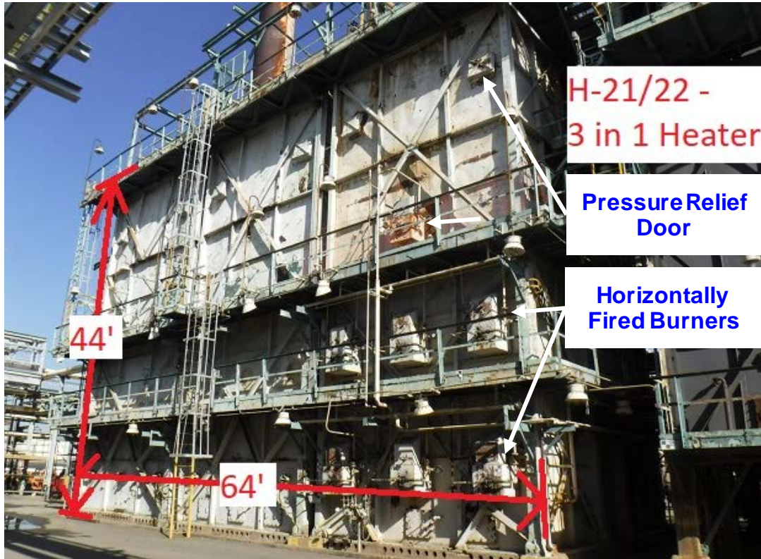
Figure 1-7 Horizontal fired "3-in-1" box heater.
