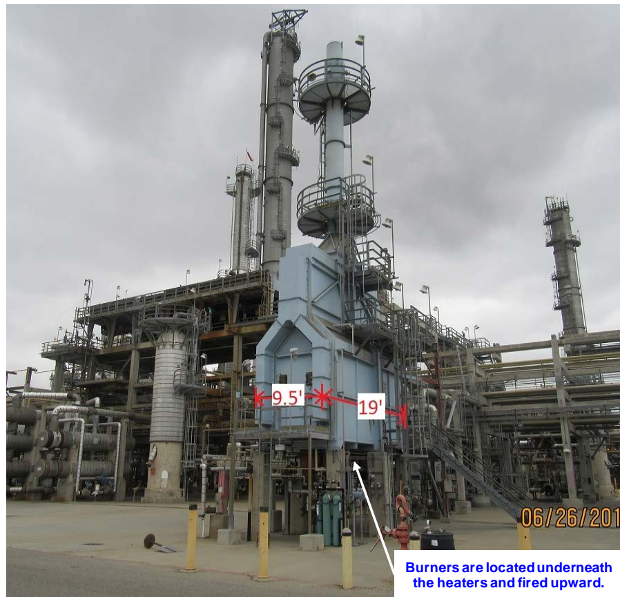
Figure 1-5 Upward fired natural draft cabin heater.
