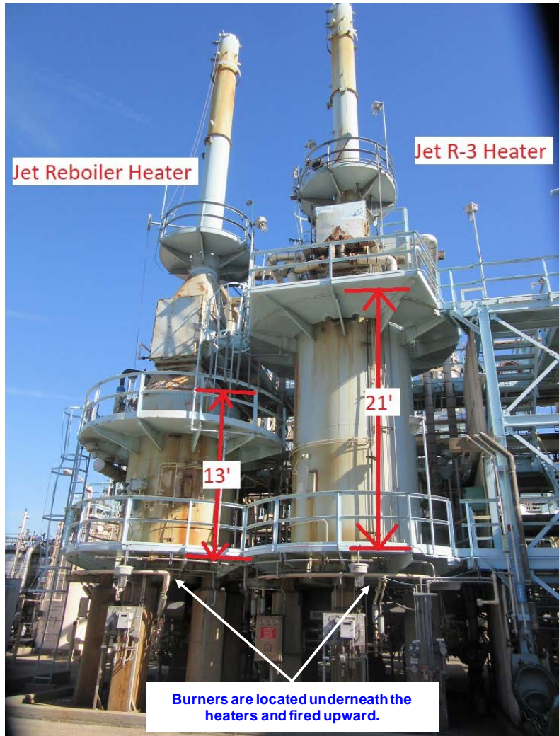
Figure 1-4 Two vertical cylindrical heater configurations.
