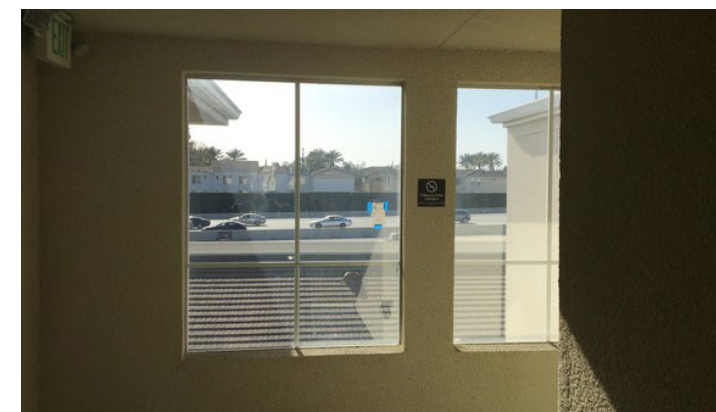
Above: view from outside the window of one UV building Source: KCRW
