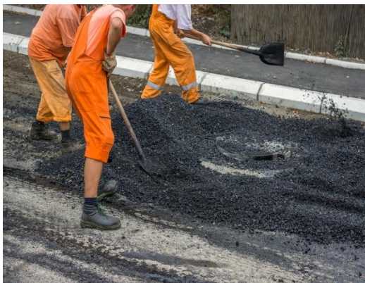
Figure 5f-2: Asphalt being used for paving
