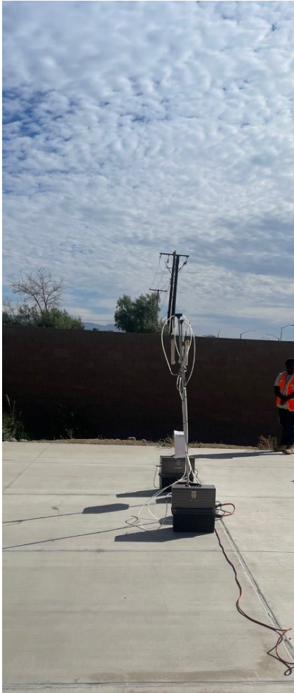
Mecca Fire Station – Facing East
