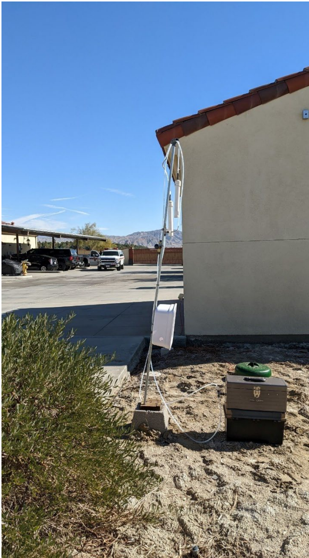
Thermal Fire Station Site – Facing East
