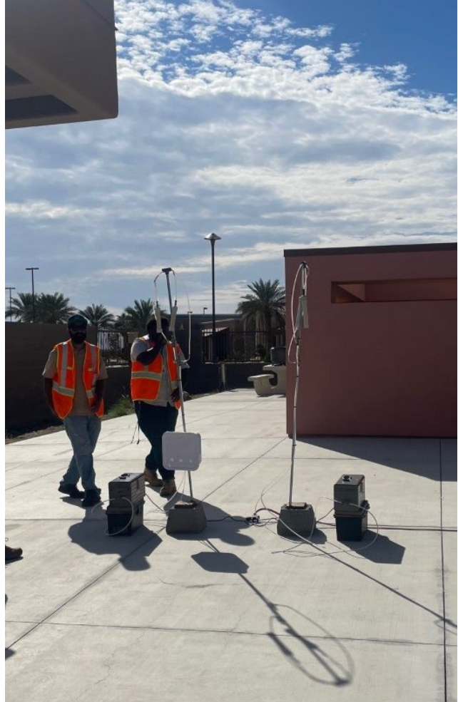
Mecca Fire Station – Facing South
