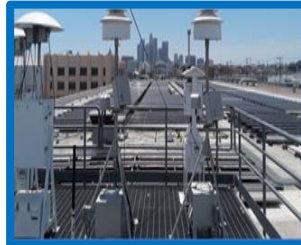
Central Los Angeles Air Monitoring Station (ELABHWC)
