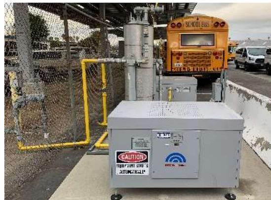
Figure 1: BRC FuelMaker FMQ-8-36
