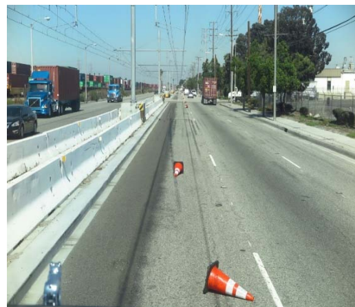
Figure 17: eHighway Infrastructure on Alameda Street
