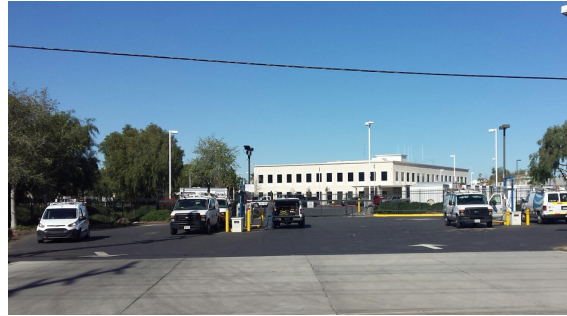
Figure 3: Station after Upgrade
