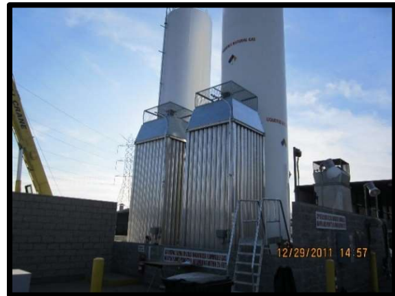
Figure 1: LNG Tank Installation
