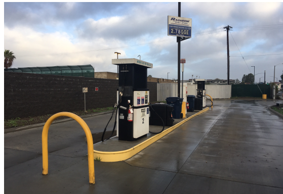
Figure 2: Public CNG Station
