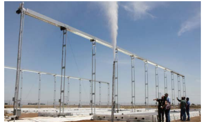
Hyperlight Solar Thermal System
